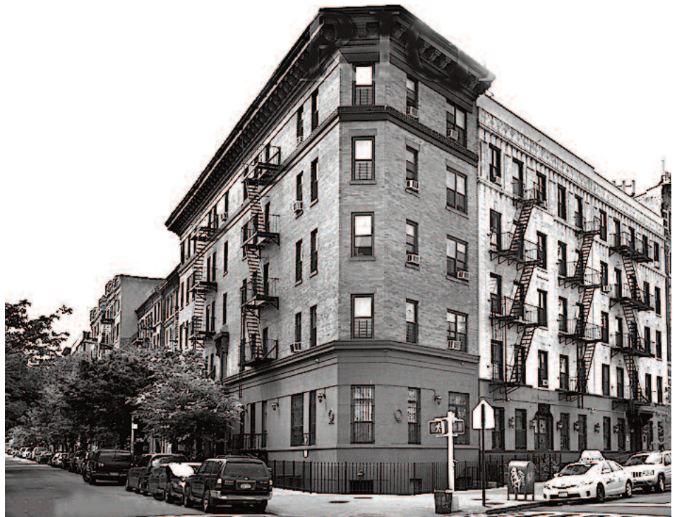
Tenants have bought the building, above, at 11-15 St. Nicholas Avenue, and one on the corner of West 11th Street, and are renovating them.
